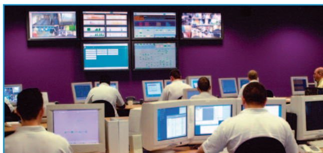
Managed Services - InTechnology's secure data centre
